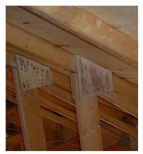
the chord and to the stud, and the type of construction adhesive to be used between the plywood gusset plates and the lumber truss members.
