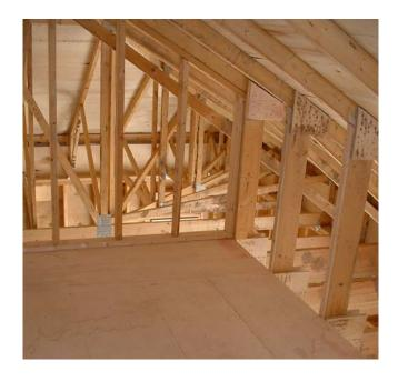
Photo 2 (below) shows the detail of the attachment of the studs for the new knee-wall. The truss manufacturer's engineer designed this arrangement, with the knee-wall studs becoming part of the truss web. The load calculations included the change in the weight of the truss itself; the dead loads (weight of the floor, gypsum board, furnace, ducts, and pipe); and live loads (weight of a serviceperson and tools).
